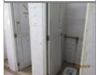
External photo(s) of the production unit(s) NO-15 Toilet with door.JPG
