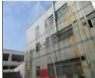
External photo(s) of the production unit(s) NO-28 Fire hydrant testing.JPG
