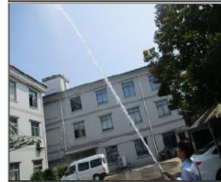
Photo of fire safety equipment The testing for fire hydrant.JPG
