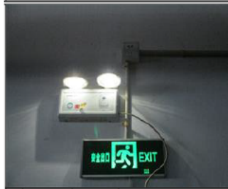
Photo of fire safety equipment The testing for emergency lights.JPG
