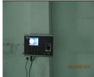
Photo of the inside of the main production hall Attendance record machine.JPG
