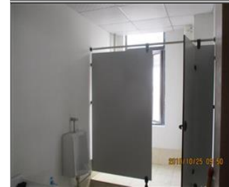
Photo of the sanitary facilities Toilet.JPG
